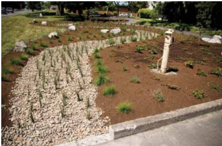
Vernier bioswale traps pollutants and silt before they enter a nearby stream
