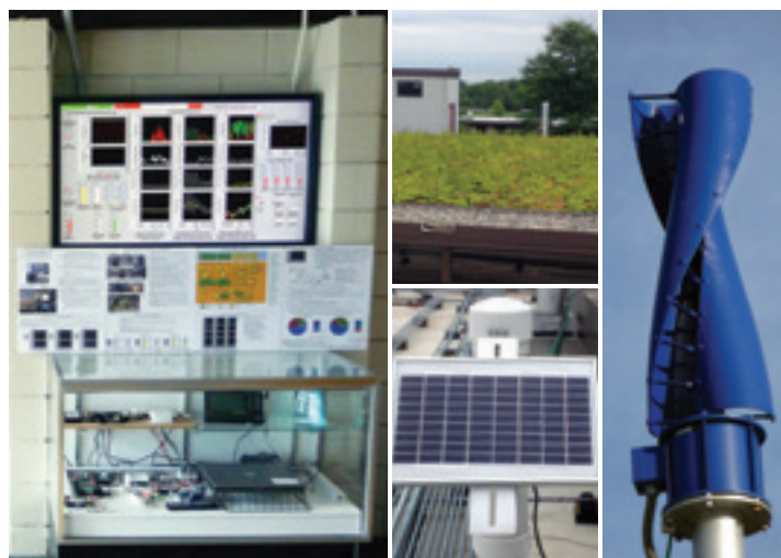
GRED dashboard displaying rooftop data from green roof, solar array, and wind turbine
